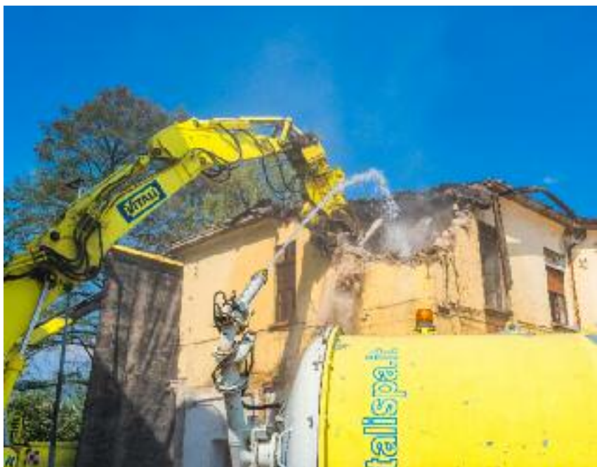
Fig. 2. Demolition with a hydraulic claw and the reduction of dust pollution.
