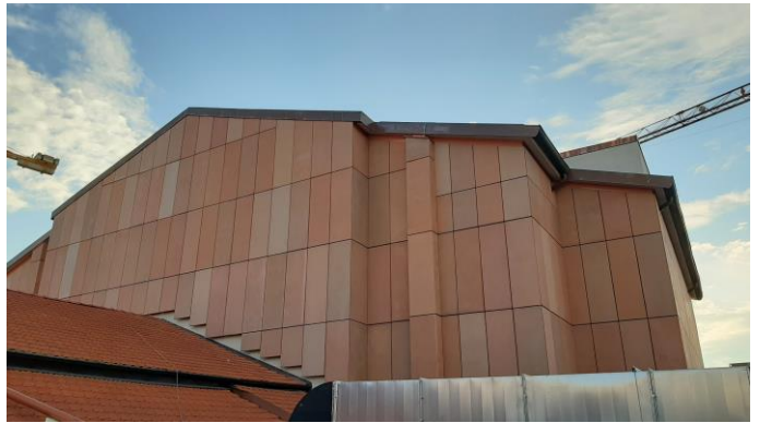
Figure 2. Northern view of the Scenic Tower. / Vista nord della torre scenica.
