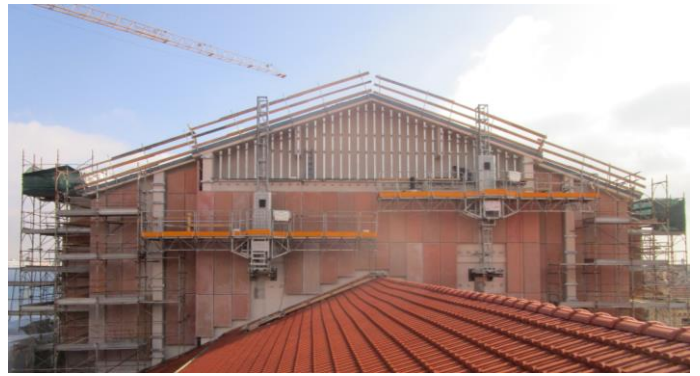
Figure 26. North Scenic Tower assembly. / Montaggio della Torre Scenica a nord.
