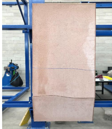
Figure 23. Cracking state of the panel. / Quadro fessurativo del pannello.
