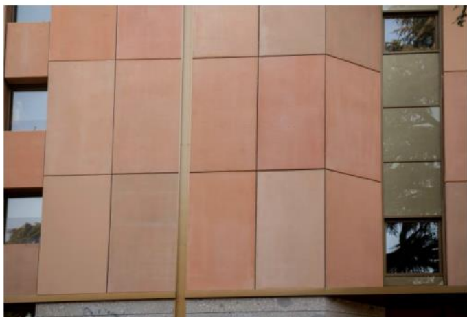
Figure 9. Cladding of the multipurpose room. / Rivestimento della sala polivalente.
