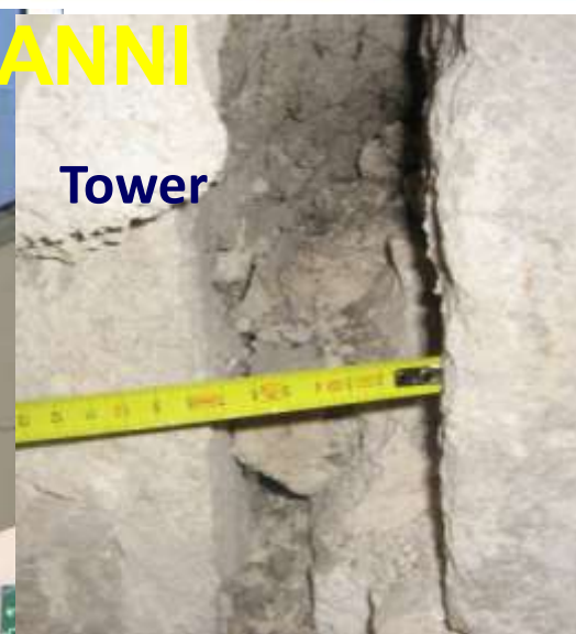
Shear collapse
