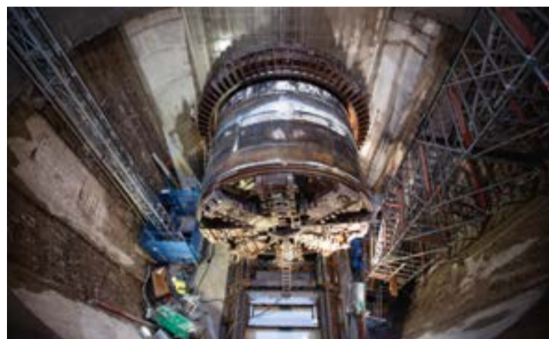
Foto 2. Breakthrough Pozzo 5.4 (© Metro C scpa)
