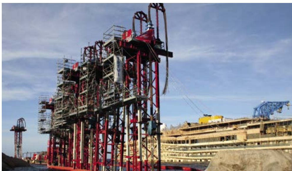
Costa Concordia recovering project. (ph. credit Trevi)
