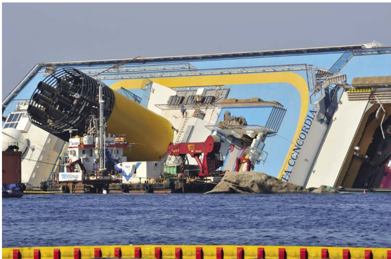
Costa Concordia recovering project. (ph. credit Trevi)
