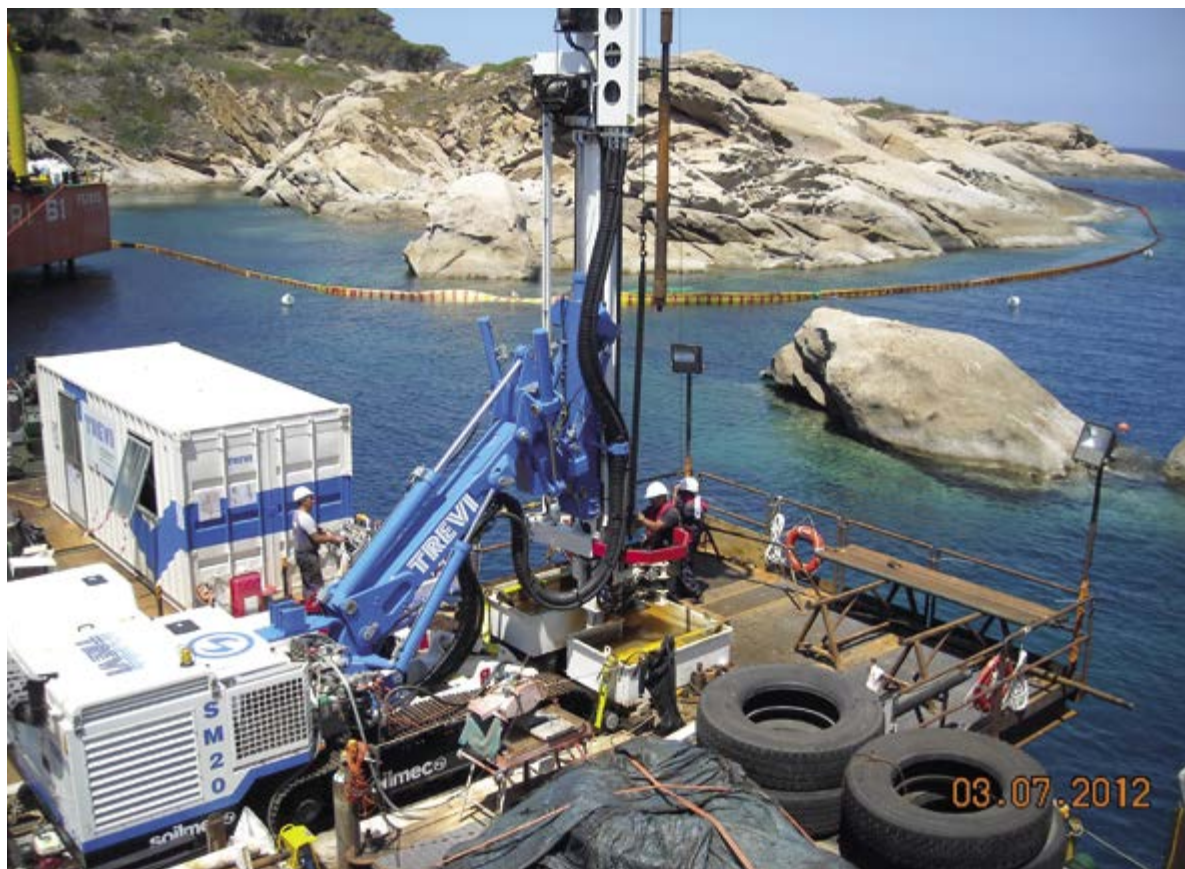
Costa Concordia recovering project. Carotaggio (ph. credit Trevi)
